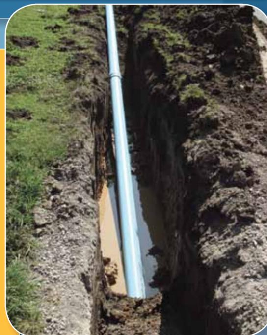
Meets AWWA C900, ASTM D1784 and UNI-B-13 Million Cycle Test.
