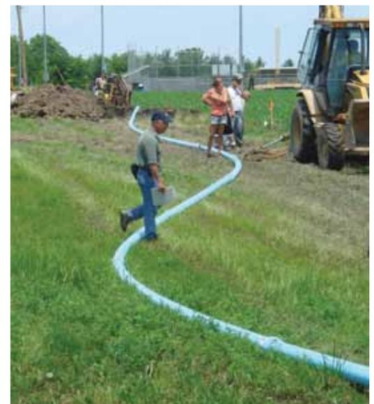
The 4-inch Eagle Loc 900 was installed in 400-foot lengths.
