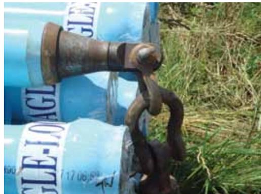
The contractor attached an 8-inch reamer directly to the pulling head and pipe.
