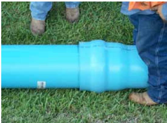
Figure 6: Assembly has just begun. The spigot has made contact with the grip ring inside the bell.
