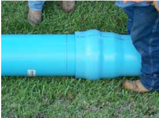
Figure 5: Assembly continues until the insertion line is even with the lip of the bell, as shown above.
