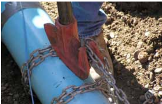
Figure 10: This assembly tool uses a chain wrapped around the bell and a lever bar to make the joint.
