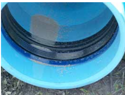
Figure 1: The sand and grit shown above must be cleaned from the internal-restraint hardware. Dirty hardware may prevent the restraint mechanism from working.
