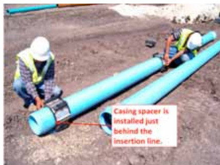
Figure 15: Casing spacers should be installed just behind the insertion line to prevent over insertion.
