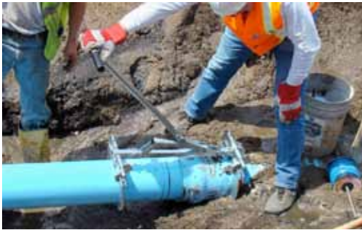
Figure 9: This assembly tool is called the Eagle Claw and is available from Pro Pipe Solutions.
