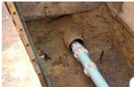
Figure 14: By using Eagle Loc, pipe may be pushed or pulled into the casing.
