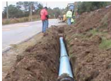
LOOKING TOWARDS THE INSERTION POINT.
