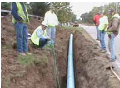
LOOKING AWAY FROM THE INSERTION POINT.
