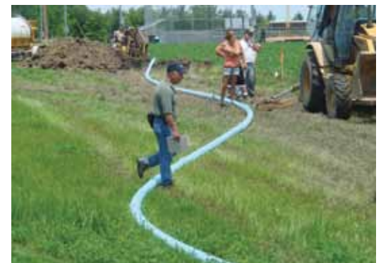
The 4-inch Eagle Loc 900 was installed in 400-foot lengths.
