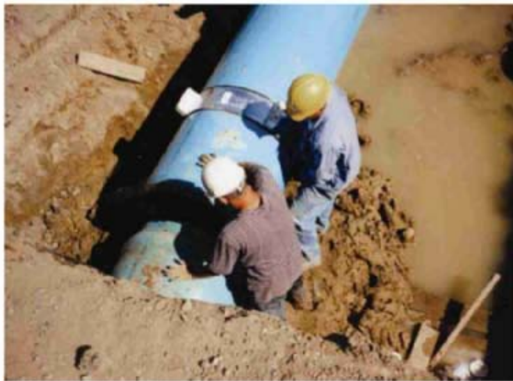
JM Eagle's new internal joint restraint, Eagle Loc 900 being installed
