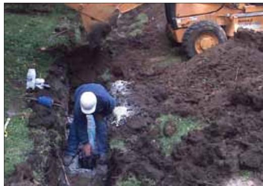
"We filled it to 300 psi and had it lying on the ground and took a back hoe to it," explains Ernie Hamilton, assistant manager of construction. "We had to hit with the tooth on the bucket to break it. It was pretty amazing. I was impressed with its strength, and particularly impressed with how it doesn't split out when outside forces damage it."
