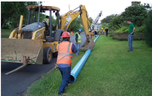
Figure 10: The backhoe's bucket center loads the previously installed length of pipe to keep it from moving while the new joint is being assembled
