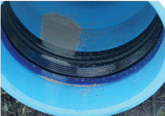
Figure 1: The sand and grit shown above must be cleaned from the restraint hardware. Dirty hardware may prevent the restraint mechanism from working.
