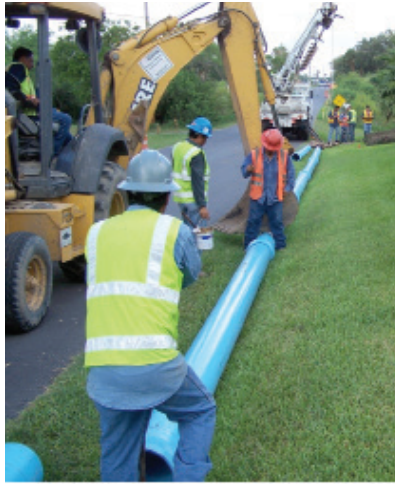
Figure 7: Example of an Eagle Loc joint assembly
