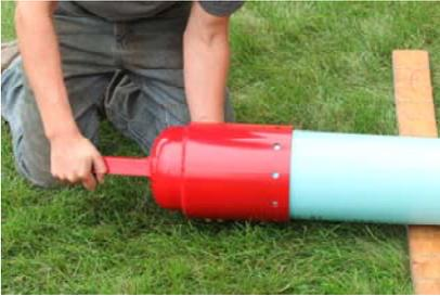
Step 2 – Install pull head over the top of the C-900 PVC pipe. Install the pull head where PVC pipe extends the end cap of the pull head.
