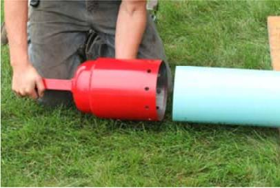
Step 1 – Align pull head with the end of the C-900 PVC pipe.
