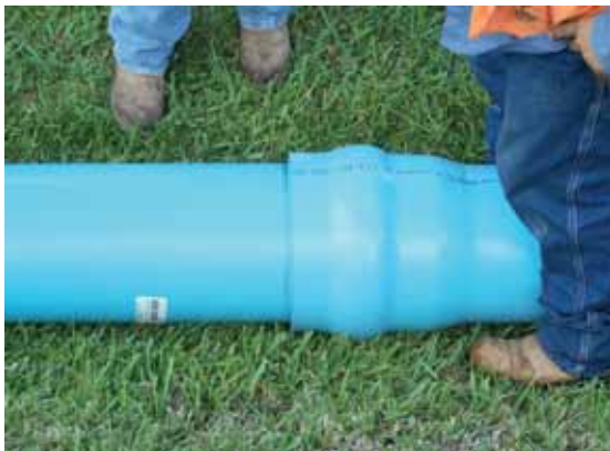
Figure 6: Assembly has just begun. The spigot has made contact with the grip ring inside the bell.
