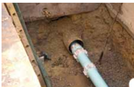
Figure 14: By using Eagle Loc, pipe may be pushed or pulled into the casing.
