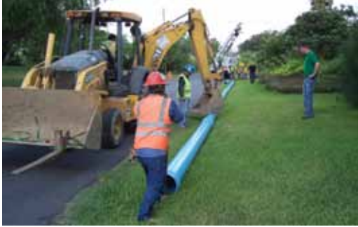
Figure 8: The backhoe's bucket center loads the previously installed length of pipe to keep it from moving while the new joint is being assembled
