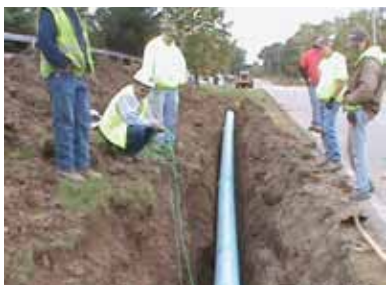
LOOKING AWAY FROM THE INSERTION POINT.
