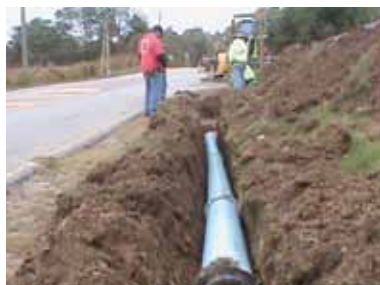
LOOKING TOWARDS THE INSERTION POINT.
