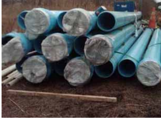
Figure 2: The shrink-wrapped ends keep dirt and other foreign material out of the bell.
