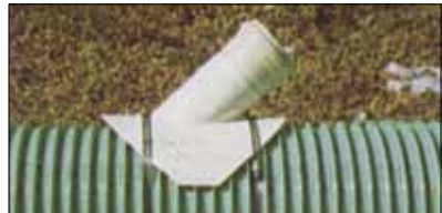
12. Attach two stainless steel bands as shown.
