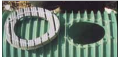
8. Properly applied silicone.
