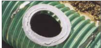
10. Apply silicone in a continuous bead as shown to the smooth side of the gasket.
