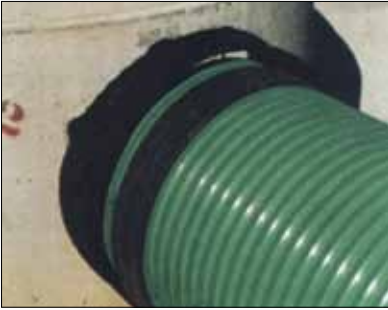
7. The pipe and gasket are ready for assembly into the manhole boot.
