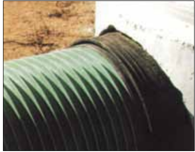
8. Position the pipe and gasket inside the manhole boot so that gasket is under the strap location.
