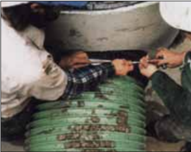
9. Tighten strap around the manhole boot with torque wrench or screwdriver. (torque to 60 inch/pounds).
