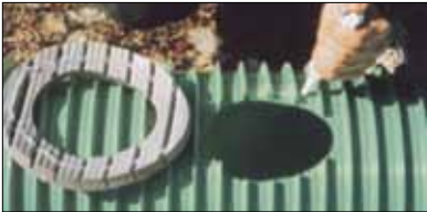
7. Apply silicone to the O.D. of Ultra Rib™ around the tap hole as shown.
