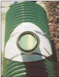
11. Properly align saddle with saddle gasket to prevent obstruction of incoming flow.
