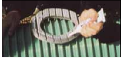
6. Apply silicone liberally around the grooved side of the gasket.
