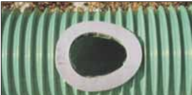
9. Place saddle gasket over the tap hole as shown.
