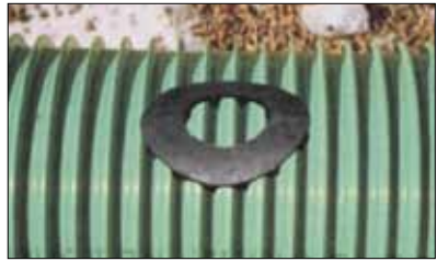
2. Place saddle gasket over the tap hole as shown.
