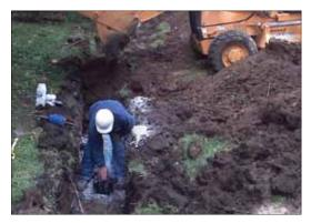
"We filled it to 300 psi and had it lying on the ground and took a back hoe to it," explains Ernie Hamilton, assistant manager of construction. "We had to hit with the tooth on the bucket to break it. It was pretty amazing. I was impressed with its strength, and particularly impressed with how it doesn't split out when outside forces damage it." McCorkendale Construction works with Water One and Superintendent Rick Lickteig is happy with Water One's choice of plastic.
