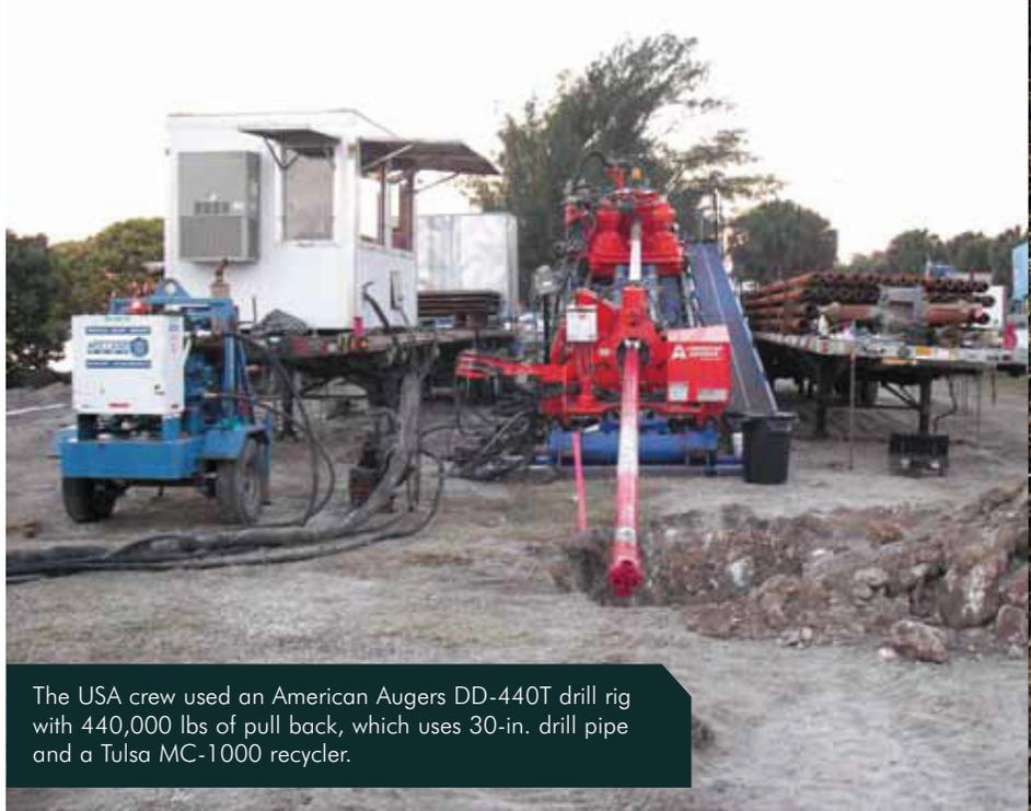
The USA crew used an American Augers DD-440T drill rig with 440,000 lbs of pull back, which uses 30-in. drill pipe and a Tulsa MC-1000 recycler.
