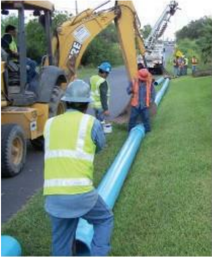
Figure 6: Example of an Eagle Loc joint assembly
