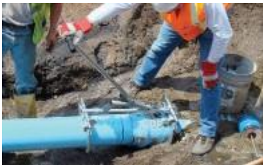
Figure 10: This assembly tool is called the Eagle Claw and is available from Pro Pipe Solutions.
